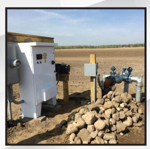
A Variable Frequency Drive (VFD) is a type of controller that varies the frequency and voltage supplied to an electric motor. Elite Industrial Mfg. (EIM)offersa turnkey, outdoor rated, custom VFD system, that designed specifically for pump and fan applications. Our "MSP" systems are designed for single phase input and three phase output, and our "MTP" systems are designed for three phase input and three phase output. Below we have added a few reasons why VFD's are beneficial in today'smarkets.
