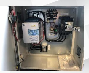
A soft starter is an electrical device used for the acceleration, deceleration, and protection of a three-phase electric induction motor. By controlling the voltage applied to the motor, we can temporarily reduce electric current surge during startup, resulting in less mechanical stress on the motor winding, shaft, power cables, and eliminate any unwanted water hammer in a pumping application. All EIM enclosed soft start packages are referred to as our WSS series.
